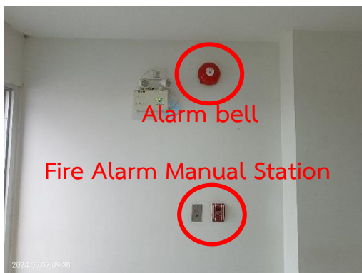
Alarm bell & Fire Alarm Manual Station
